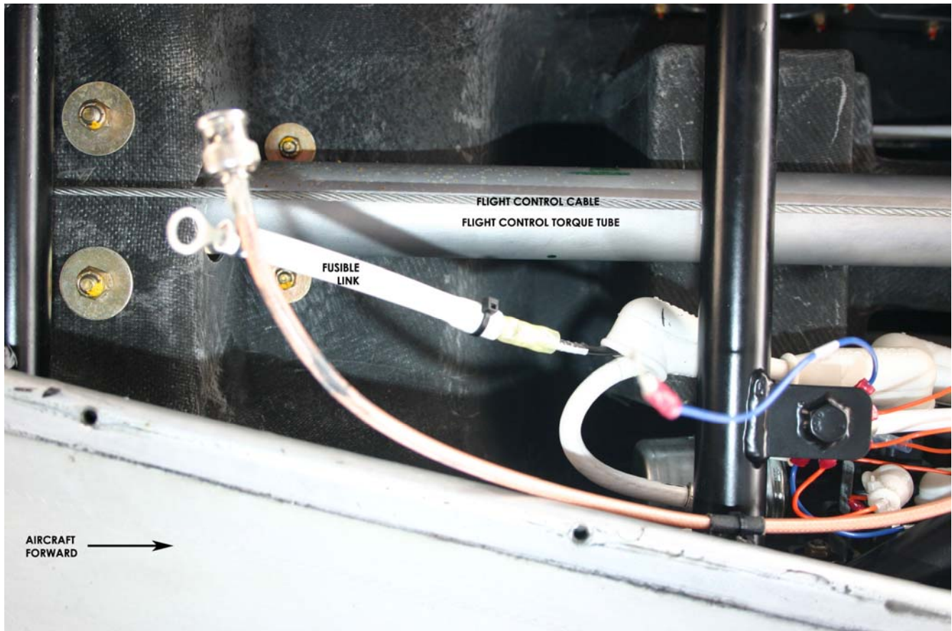
Figure 6 - Fusible Link Spliced on P03A10BK
